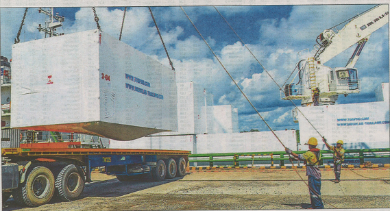
One of the modules offloaded from a container ship at the Kiunga port before being transported to the hotel site. – Picture courtesy of OTDF
